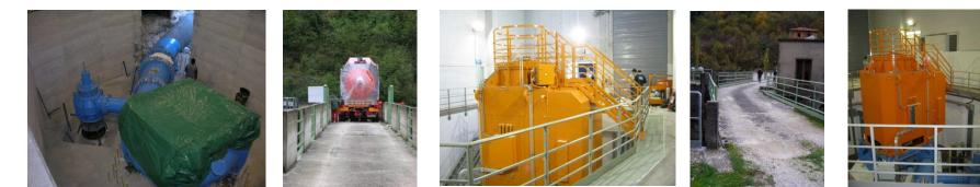
Turbine Generator Inlet valve Governor System Electrical equipment Erection and commissioning Main and Aux Transformers Turbine type: Vertical Francis Net Head: 152.6 m Flow rate: 4.04 mc/s Output: 1x 5443 kW Speed: 750 rpm Year: 2008 Country: Italy
